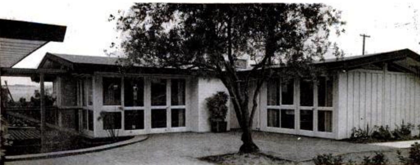
Adjoining studs at ends of panels form post to support roof. Below, home made of same panels as model has different look
